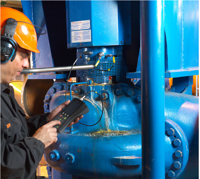
Vibration measurements in progress
